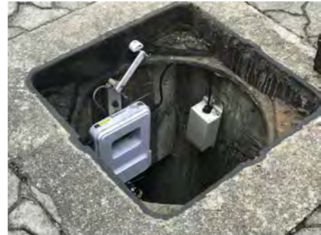
Wireless underground devices installed in manholes 於沙井安裝的無線探測裝置
